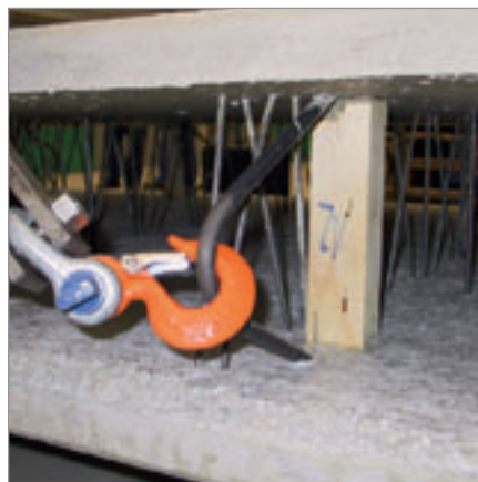
Installed KE transport anchor
