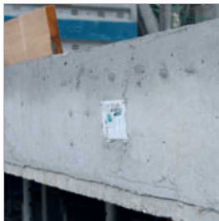
Installed sliding sleeve for HED shear dowel
