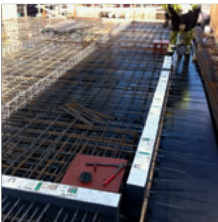
ISOMAXX® elements being fitted on the building site
