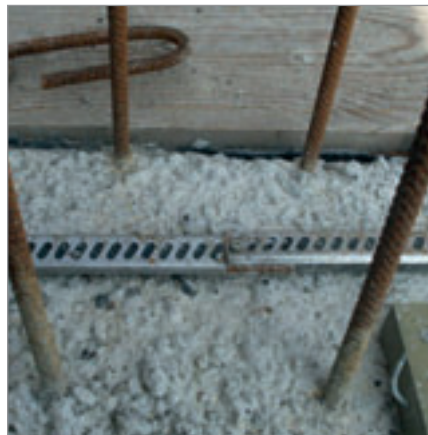
Fastening of SWELLFLEX® swelling tape with a metal channel
