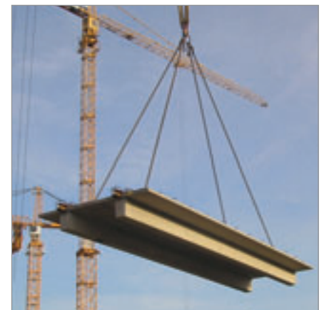
Transport of a TT plate with PFEIFER Steel Bearings
