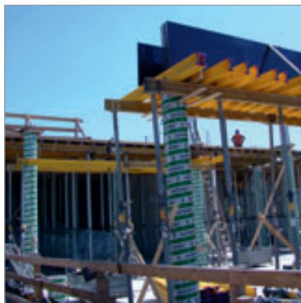
RAPIDOBAT® shuttering tubes on the building site
