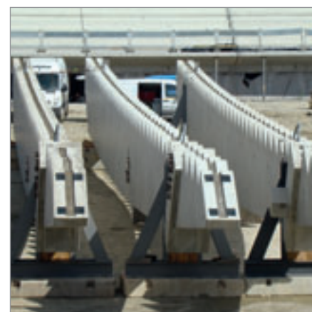
Raker beams with PFEIFER BS Anchors ready for transport
