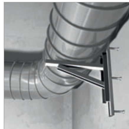
Fastening pipes and media carriers
