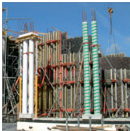
RAPIDOBAT® lined; on the left already removed
