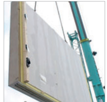
Prefabricated wooden wall with POWERCON® and ENERCON® connectors
