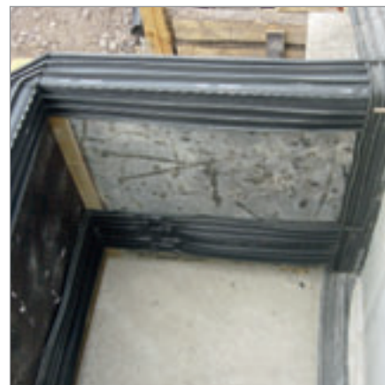
Sealing of a construction joint with KUNEX® waterstop-corner joint
