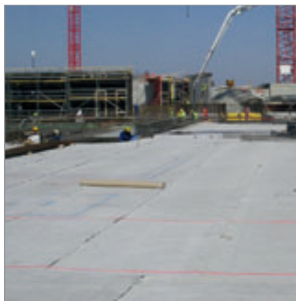
Surface sealing with SWELLPROOF DS
