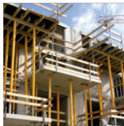
Prefabricated balcony connected using ISOPRO® elements
