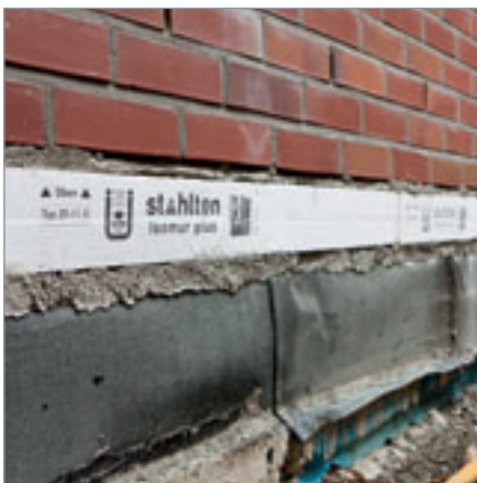
ISOMUR® wall base elements in combination with facing brickwork
