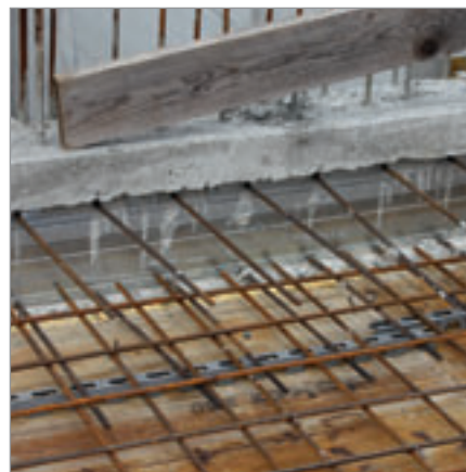
FERBOX® rebending connection type B set in concrete on wall; for connection to a ceiling
