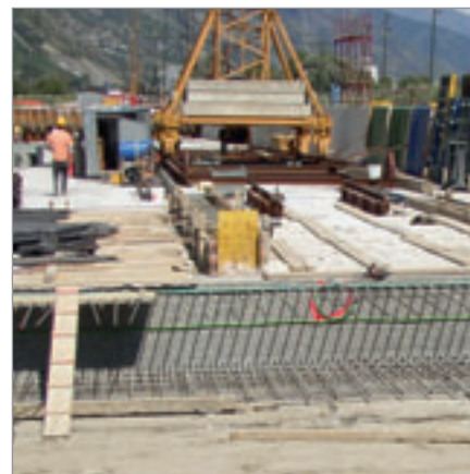
Joint sealing with PLURAFLEX® injection hose
