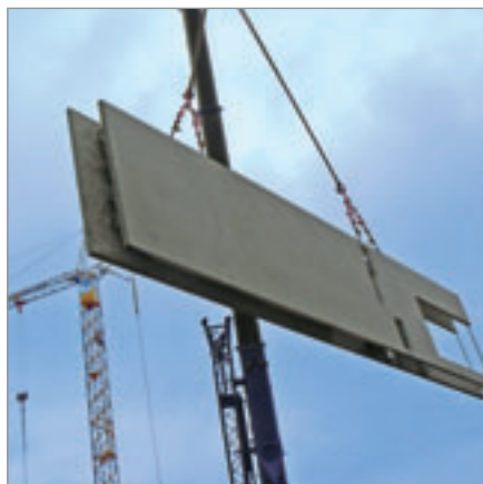
Moving an element wall using KE transport anchor
