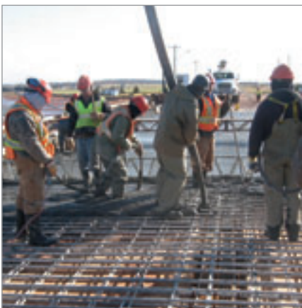
Bridge reinforcement with FIBERNOX® V-ROD
