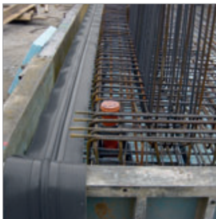
Sealing of an expansion joint with KUNEX® expansions joint tape
