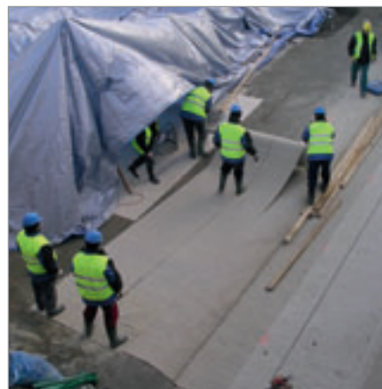
Surface sealing with SWELLPROOF bentonite sealing mat
