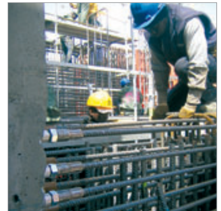
Connection of a precast concrete column to a cast-in-situ joist
