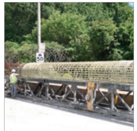
Column reinforcement with FIBERNOX® V-ROD
