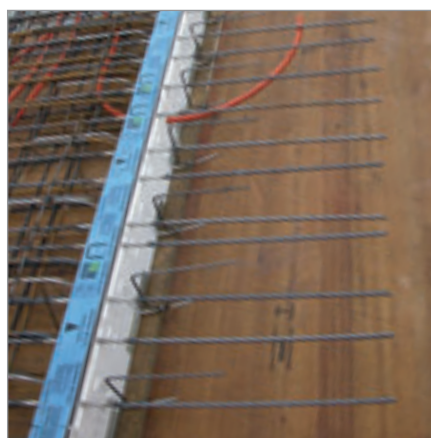
ISOPRO® elements during reinforcement work
