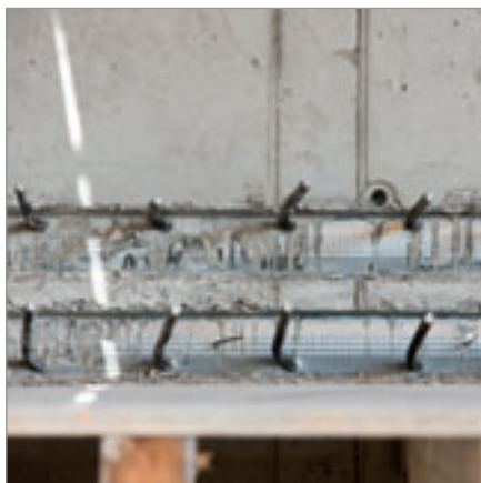
FERBOX® rebending connection type D with reversed reinforcing beams
