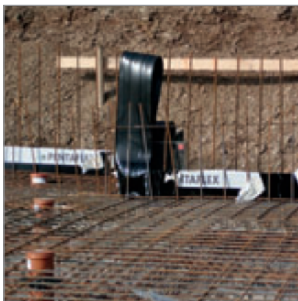
PENTAFLEX KB® joint sheet, DFA expansion joint connection and floor lead-throughs
