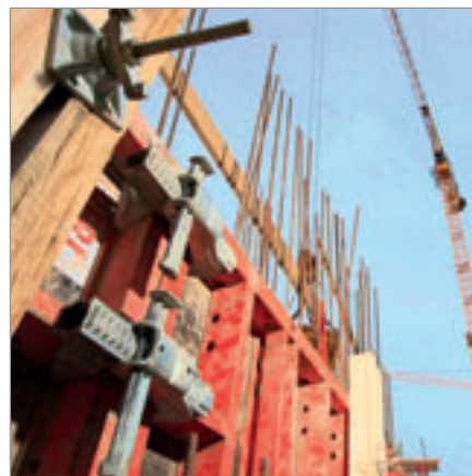
Use of anchors and formwork accessories on building site
