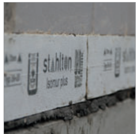
ISOMUR® wall base elements in combination with KS masonry
