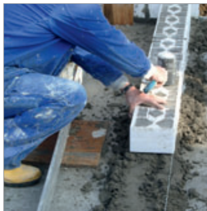
Positioning of ISOMUR® elements on the building site
