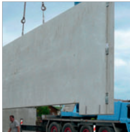
Connection of fully prefabricated parts using POWERCON®
