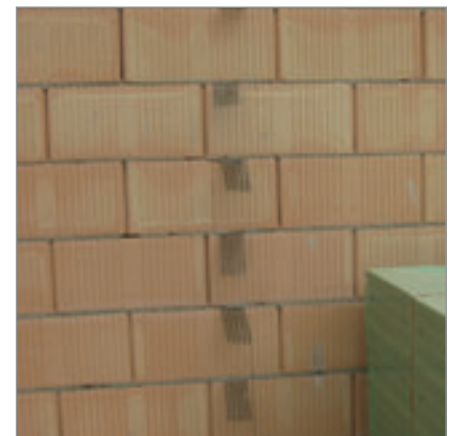
Masonry with GRIPRIP® type S
