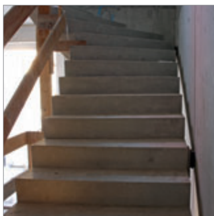
Spiral staircase with ISODORN HQW sound insulation
