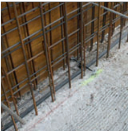
Sealing of a construction joint with SWELLFLEX® BT
