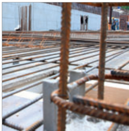
Fibre concrete spacers with vertical and horizontal reinforcement
