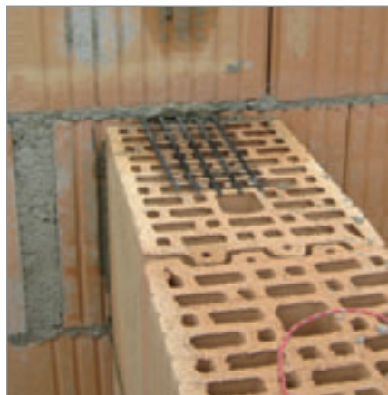
GRIPRIP® type S with masonry to be connected
