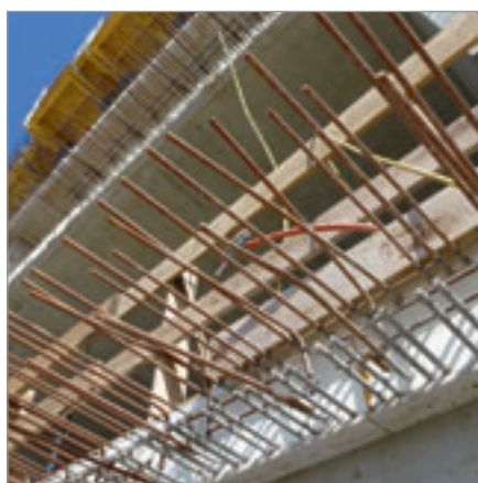
ISOPRO® elements fully mounted in the ceiling
