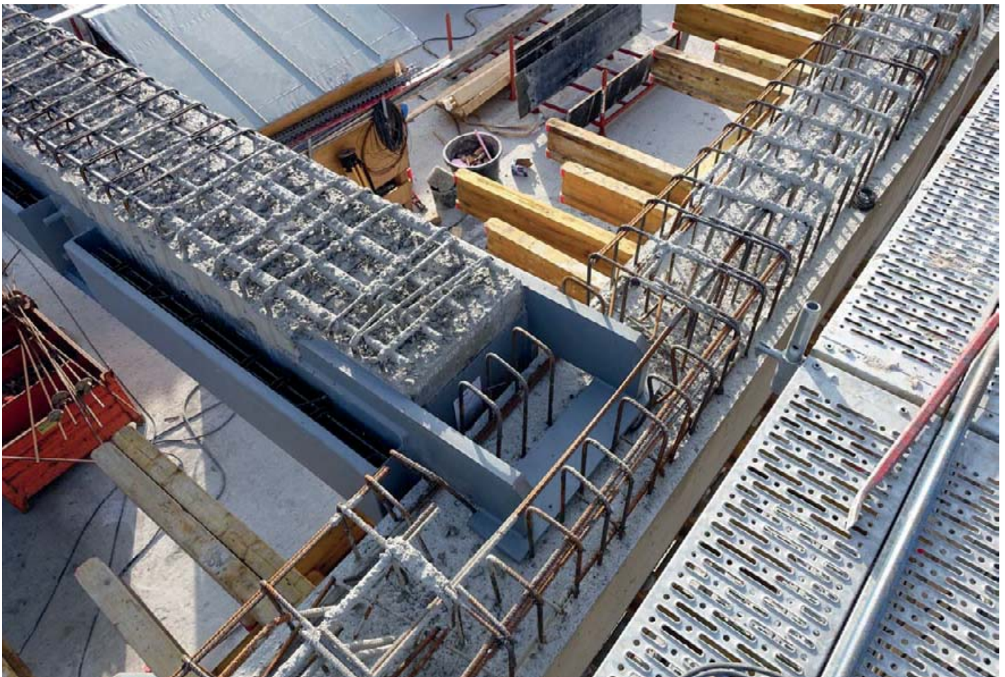
A - Technology of filling the joints with low-shrink mortar
