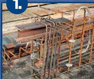
Installation of reinforcement
