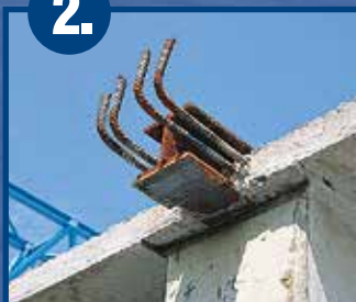
Installation in precast concrete elements
