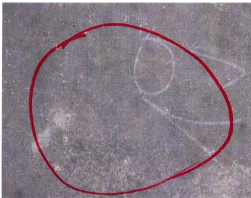
Fig. 5 Detail – undamaged outside surface of test specimen A – anchor 1
