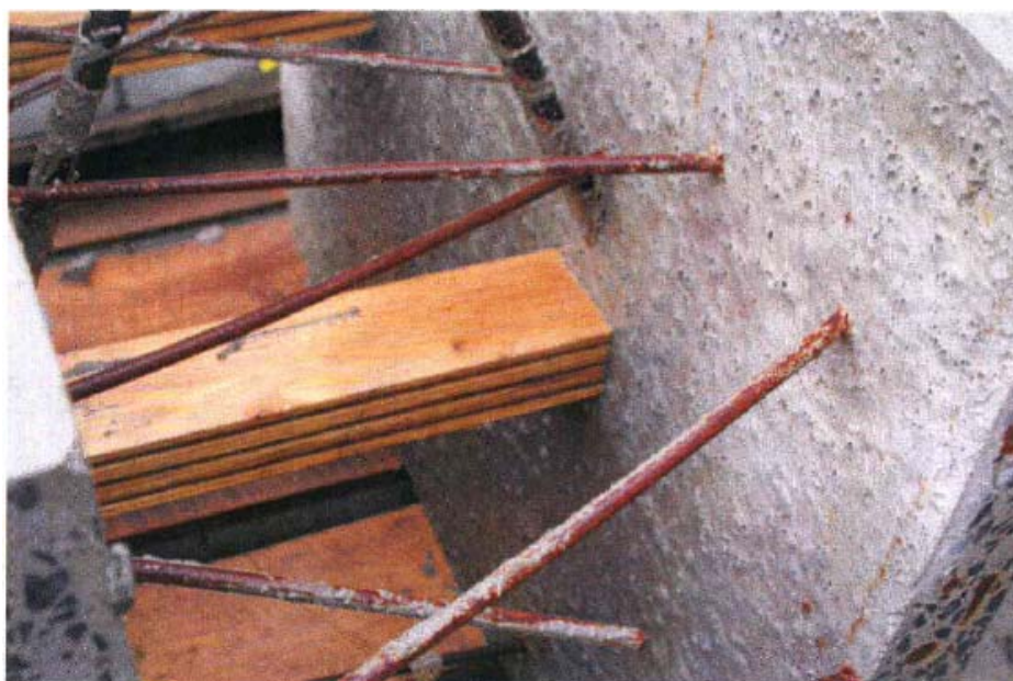
Fig. 2 Detail of test specimen A
