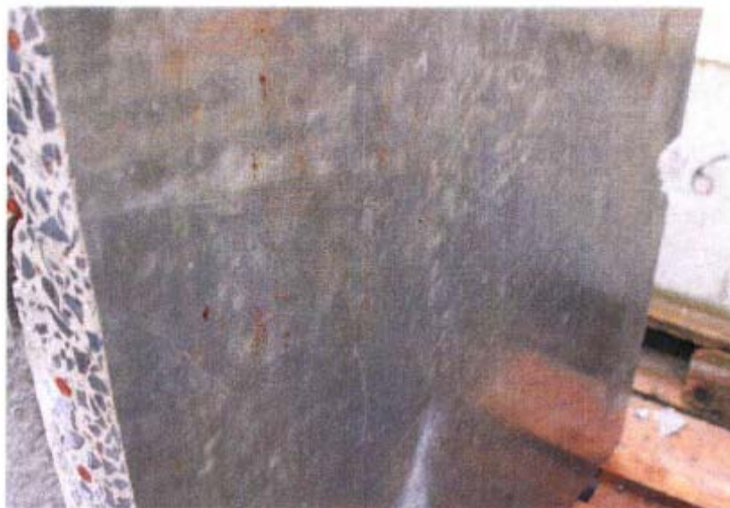
Fig. 3 Outside surface of test specimen A
