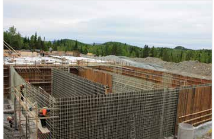
Tanks for sewerage treatment plant, slab- and wall reinforcement
