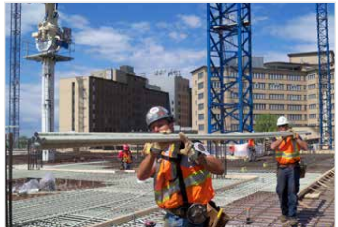
FIBERNOX® V-ROD as a non-conductive ground slab reinforcement for hospital construction
