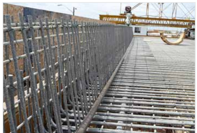
Installation of FIBERNOX® V-ROD in bridge deck and concrete barrier wall
